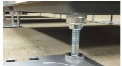
Step 1 and 3: loosen and fasten the pedestal at the lock-nut at bottom
