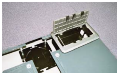
Cables extending from Cable Trenches to wall base, desktop, any point of the workstation
