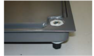
Socket-Set-Crew Fixed at top of the pedestal
