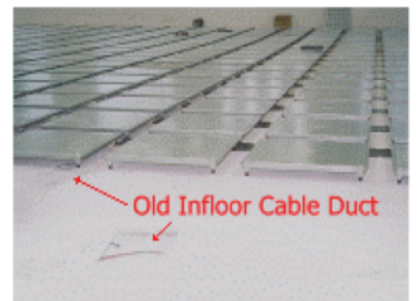
Renovation jobs: Installing on the old, embed floor trenches
