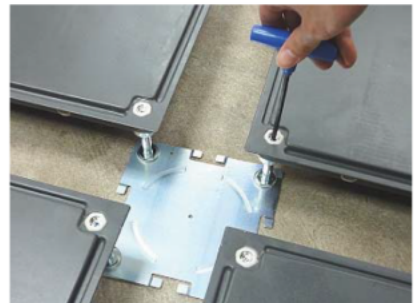
Step 2: adjust height from top by key wrench
