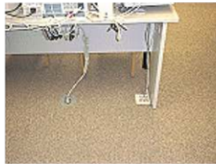
Extension through Exit-Cap to desk top or workstation
