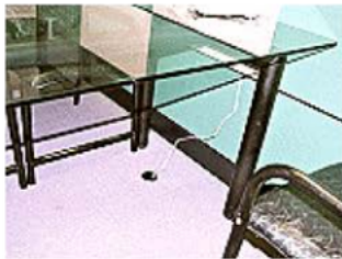
Extension through Exit-Cap to desk top or workstation
