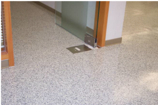
Meeting room door hinge installed on AN45 panels
